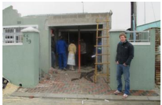
Construction for the first floor has begun.
