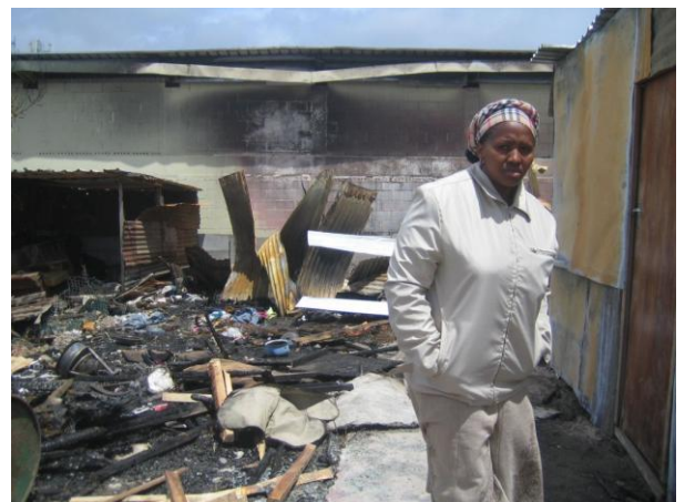
..... after the fire.
